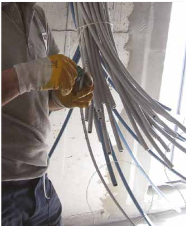
An operator stripping cables during installation.
