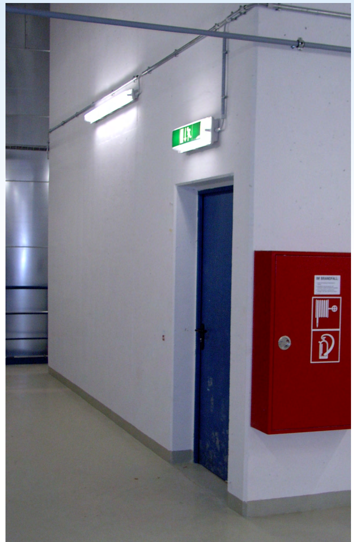
Integration of emergency luminaires with self-contained batteries - Emergency luminaires can be used with the following three types of circuit: Continuous light, standby light and controlled light.
