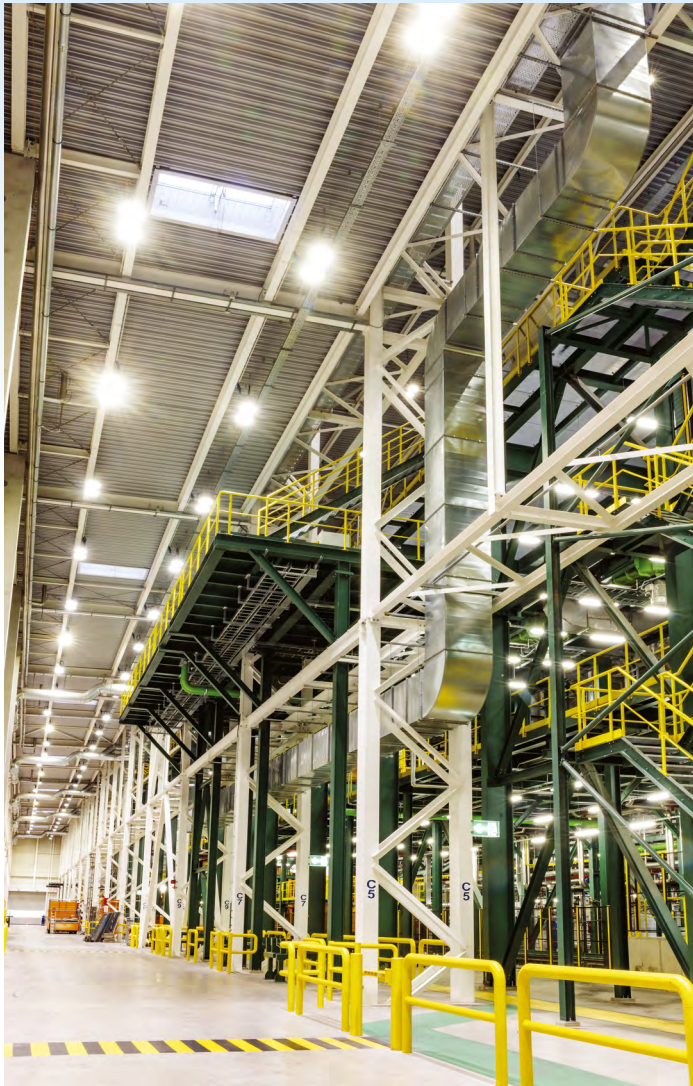
High Bay light fittings control by using the calendar function - In addition to full days, time-specific settings can also be selected. It makes sense if e.g. the complete lighting should be switched to 100% in a company during core working hours.
